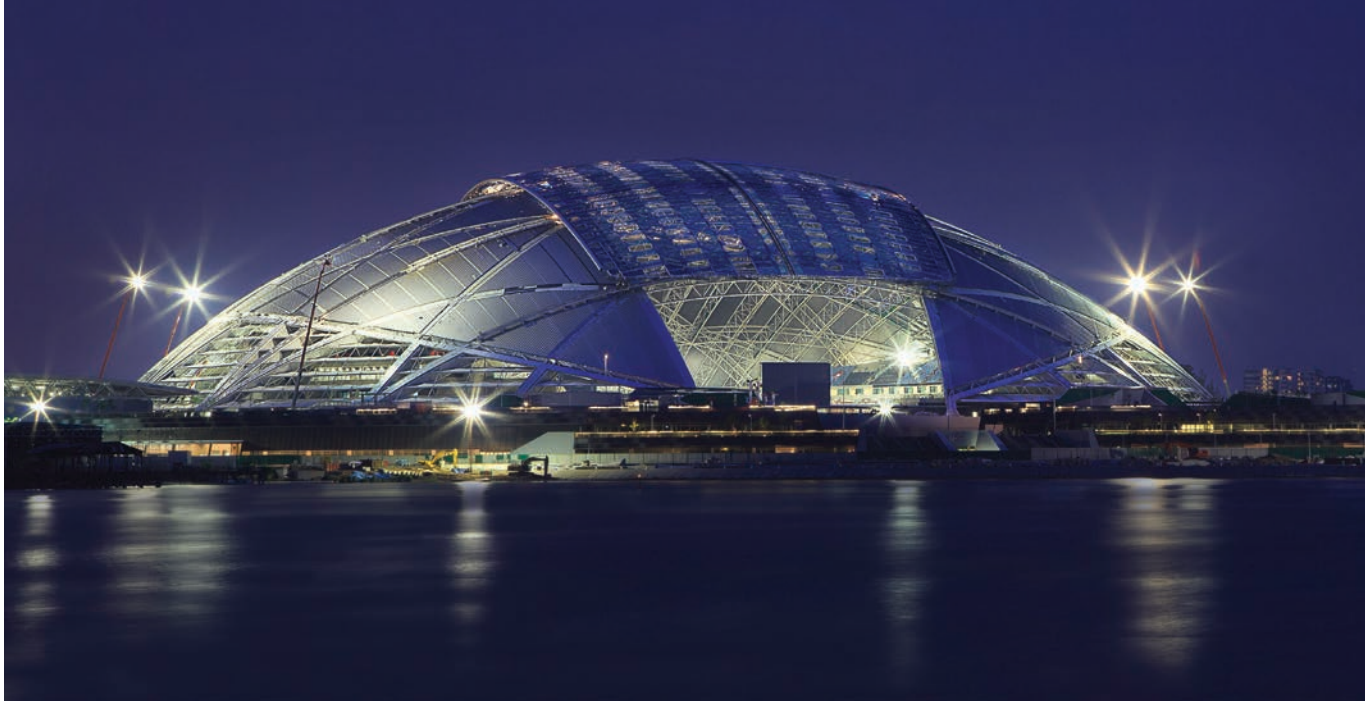
Curved in two directions, the Singapore Stadium roof moves with a hoisting system that must accommodate the shape of the structure, the weight of the roof and the wind load. This picture shows the roof closing for the first time on April 15, 2014. Photo by Stanley Cheah
