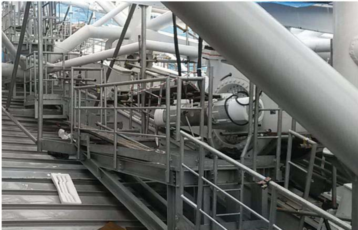
Figure 26: Drive unit – Catwalk for access and maintenance.
