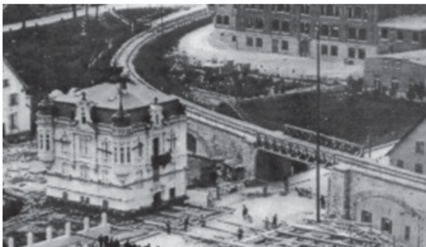
Figure 2: Relocation of Villa Haux at Ebingen.
