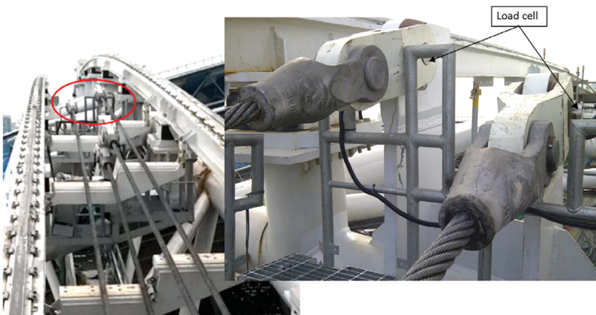
Figure 28: Wire ropes anchoring.
