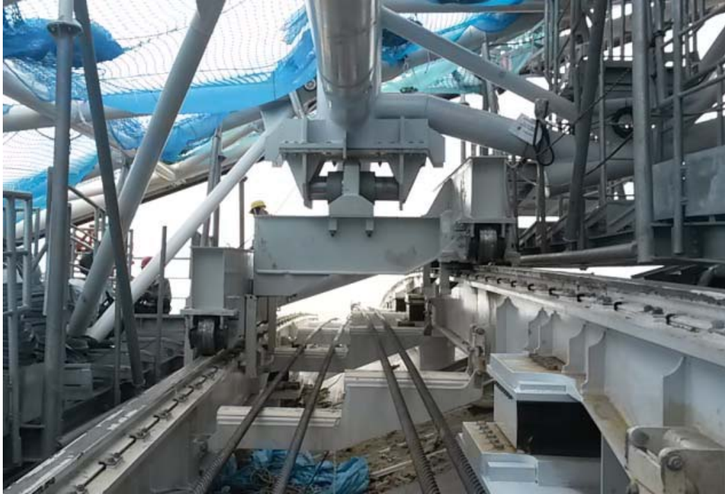
Figure 27: Path of the wire ropes toward the anchoring points.
